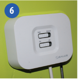
6 Securely screw the front of the receiver in place.
